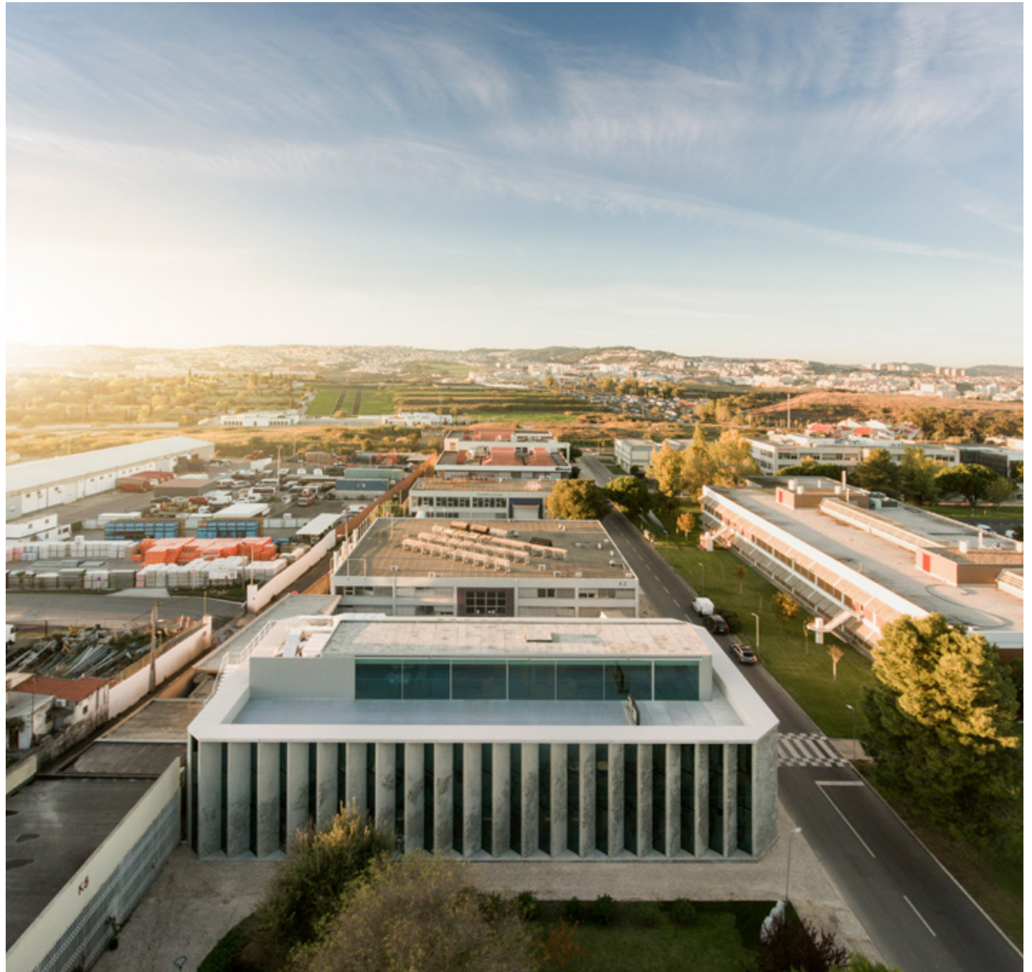
Untitled, 2016 Centre for Innovation and Competitiveness | GS1 Portugal headquarters Precast concrete moulding 49 panels, each 778 × 137 × 30 cm
